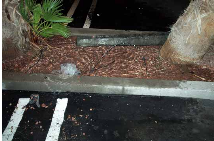
Regular reviews of your drip system can help prevent water waste.
